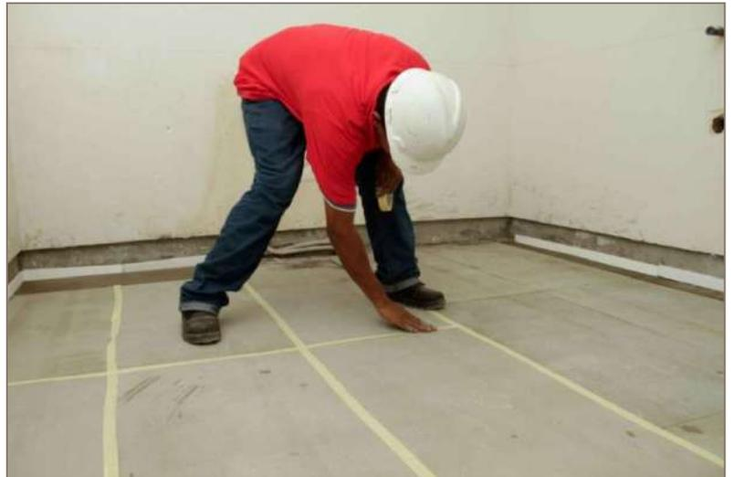
Seams are taped off, ready for the floor heating system to be installed.
