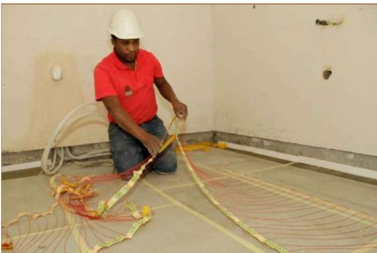
Floor heating is installed on top of the KlimaBoard insulation boards.
