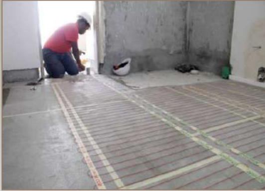
1. Heating element is unrolled on top of floor insulation and taped down.
