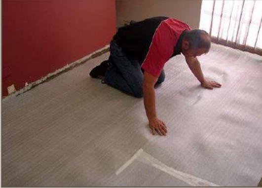
1. Foam underlay is normally installed by flooring company.
