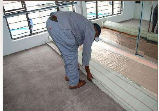
4. Carpet installation is completed.
