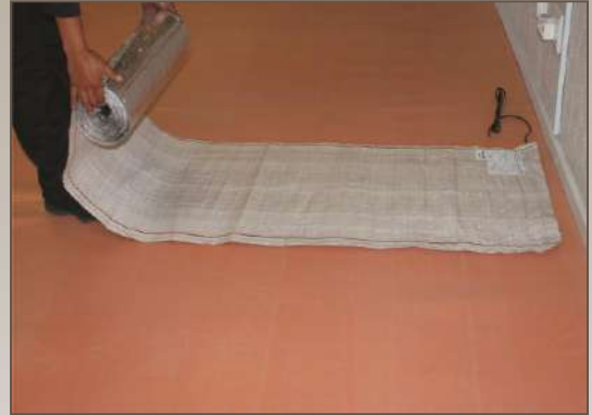
2. The carpet heater is unrolled on top of the underlay.
